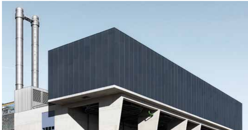
Waste Incineration Facility Winterthur
